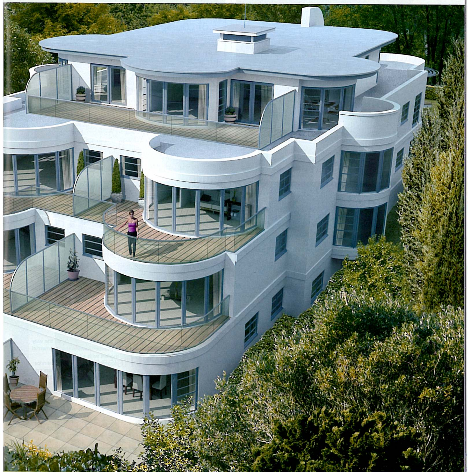
: Brooklyn House, comprising 11 luxury apartments in Bingham Avenue, Poole, Dorset. The walls have been constructed using Insulating Concrete Forms from ICF Tech, a supply and fit ICF system.
